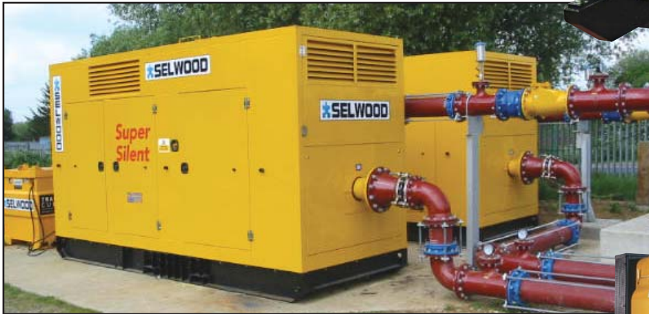
Flushing and priming of transfer main (UK)
